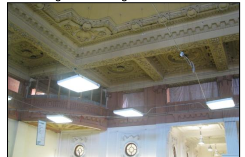
Inside, the ugly false ceiling has been removed, revealing the original ornate plaster ceiling. The light fixtures remain, for now. For more details on the current construction project, including slide shows of the work, go to http://bit.ly/9ZBps1 .
