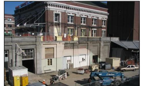
Above, the enclosure for the stairs and escalators to Jackson St. has been removed, along with the stairs and escalators. This was not a part of the original station. The open stairway build as part of the original building will be restored.
